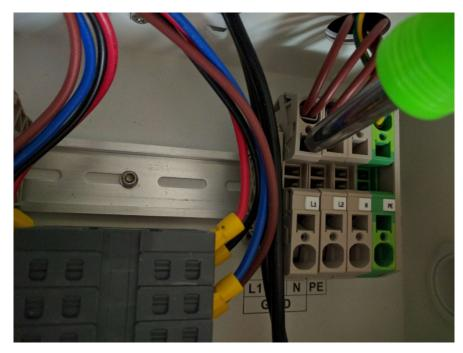
Once the screwdriver is inserted, remove the AC wire.
