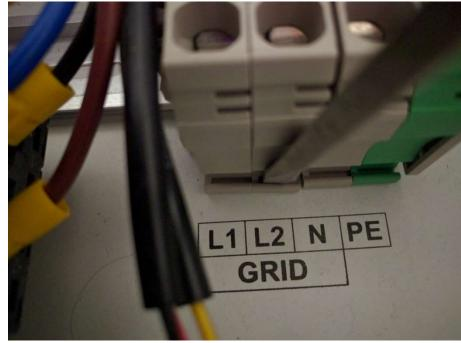
Once the latch has been released, the spring terminal will pivot off the DIN rail
