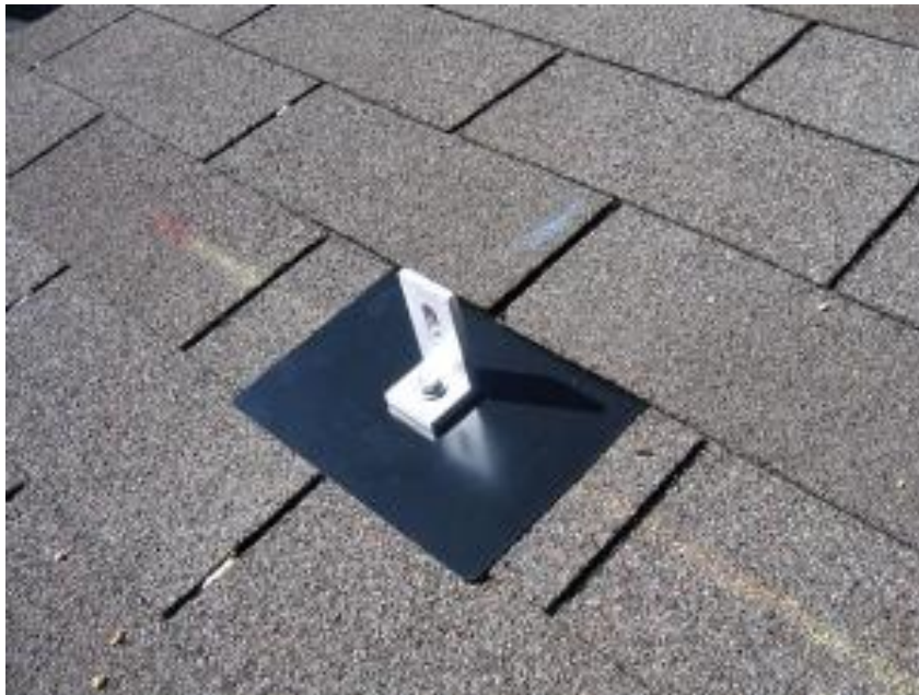
Figure 2. Flashed mounting plate with L-Foot
