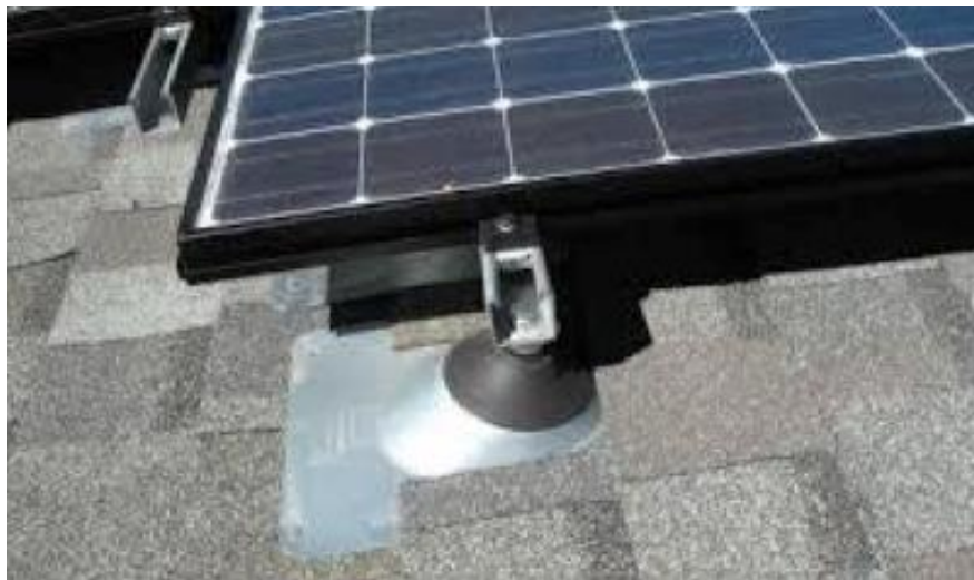
Figure 3. Flashed mounting base with Uni-Strut supporting PV modules on the Roof
