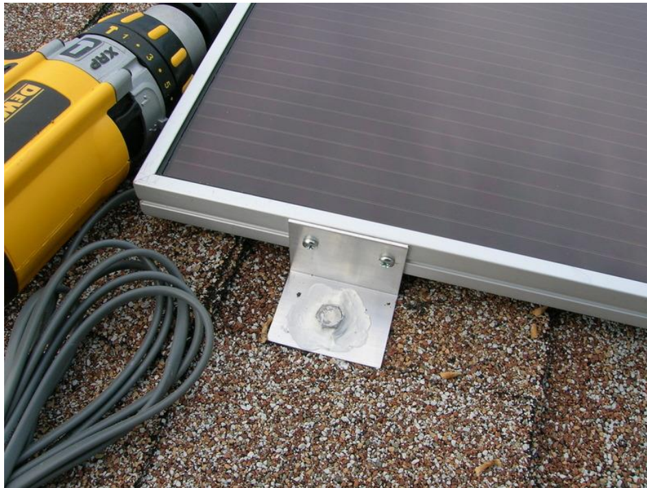
Figure 4. Un-flashed mounting base ("L-foot") sealed with silicone in the field (not recommended)
